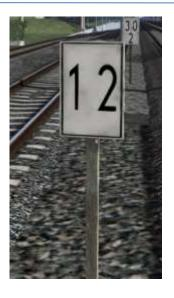
Ne 2 "Approach signal board": marking of the location of an approach signal.
